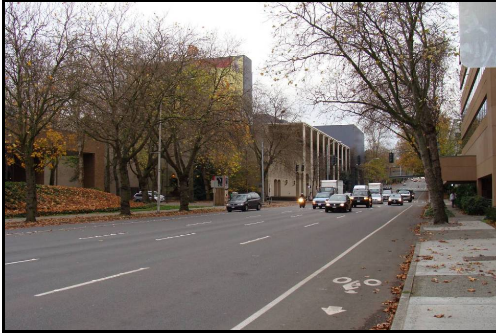
Figure 18. Viewing West on Mercer Street- KCTS building in the left foreground and the Mercer Arena in the middle ground (HRA, Nov. 14, 2008).
