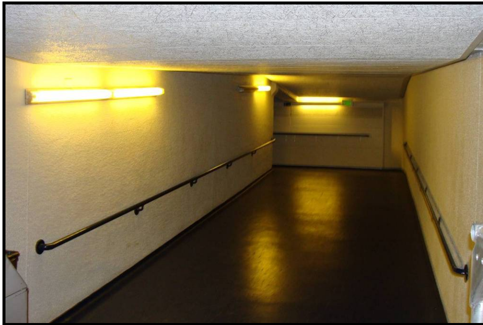
Figure 33. Viewing west from interior circulation ramps, showing wall finishes and drop ceiling added in 1964 (HRA, Nov. 6, 2008).
