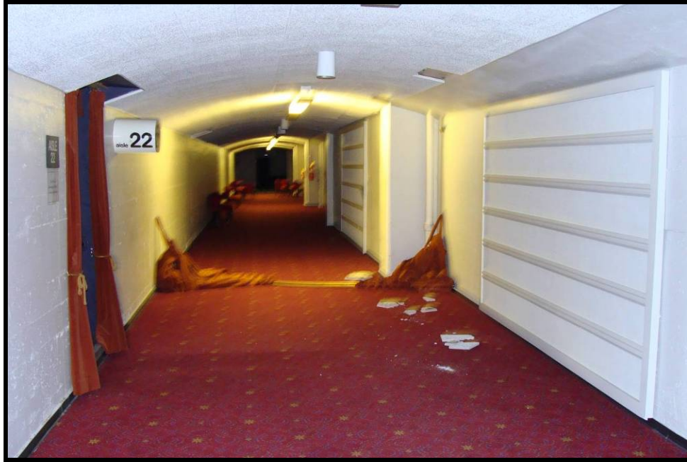
Figure 34. Viewing south from upper west corridor public area, showing acoustical wall panels and drop ceiling added in 1964. The carpet was added in 2001. (HRA, Nov. 6, 2008).
