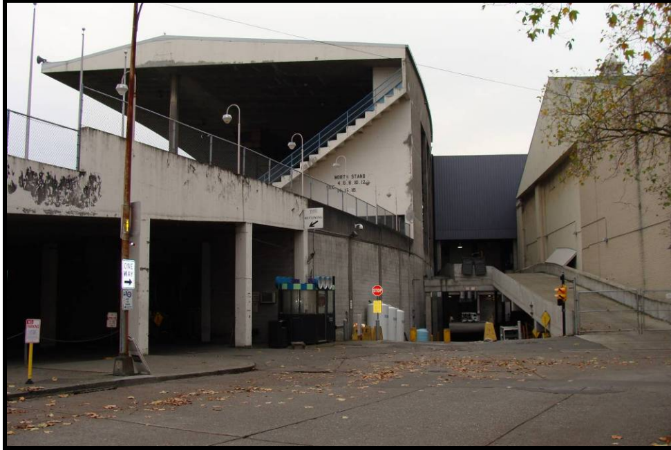
Figure 26. Viewing west. Memorial Stadium is on the left, McCaw Hall is in the middle ground. Contemporary truck loading ramp partially obscures the south façade of Mercer Arena on the right. (HRA, Nov. 14, 2008).
