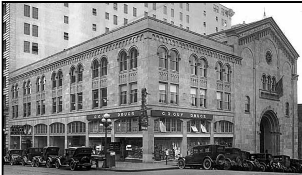
Figure 7. Chamber of Commerce Building, Seattle, Daniel R. Huntington, with Schack, Young & Meyers, Architects, ca. 1925. Source: MOHAI collections http://content.lib.washington.edu/u/?i/mlsmohai.4071
