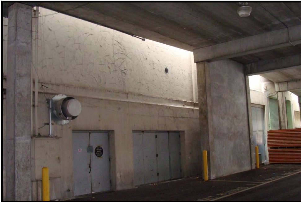
Figure 27. Loading bays on the south elevation (HRA, Nov. 6, 2008).
